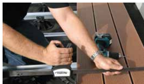
Example of application tension clamp
