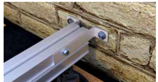
Example of application EVO wall-connection bracket
