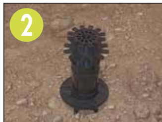
2 Once the ground anchor has been fully driven into the ground, position the adjustable pedestal onto the head plate.
