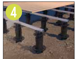
4 Finally, continue with the standard assembly of the terrace substructure – done!
