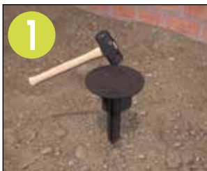
1 Drive the ground anchor into the ground using a hammer.
