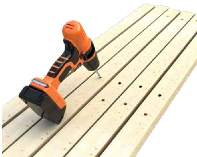
The support battens are placed on the insulation for installation. The masonry / concrete drill bit can be guided through the pre-drilled hole to pre-drill the insulation material and the substrate.
