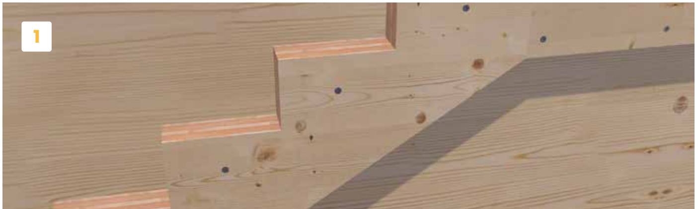
Attach the stair tread support to the wall.
