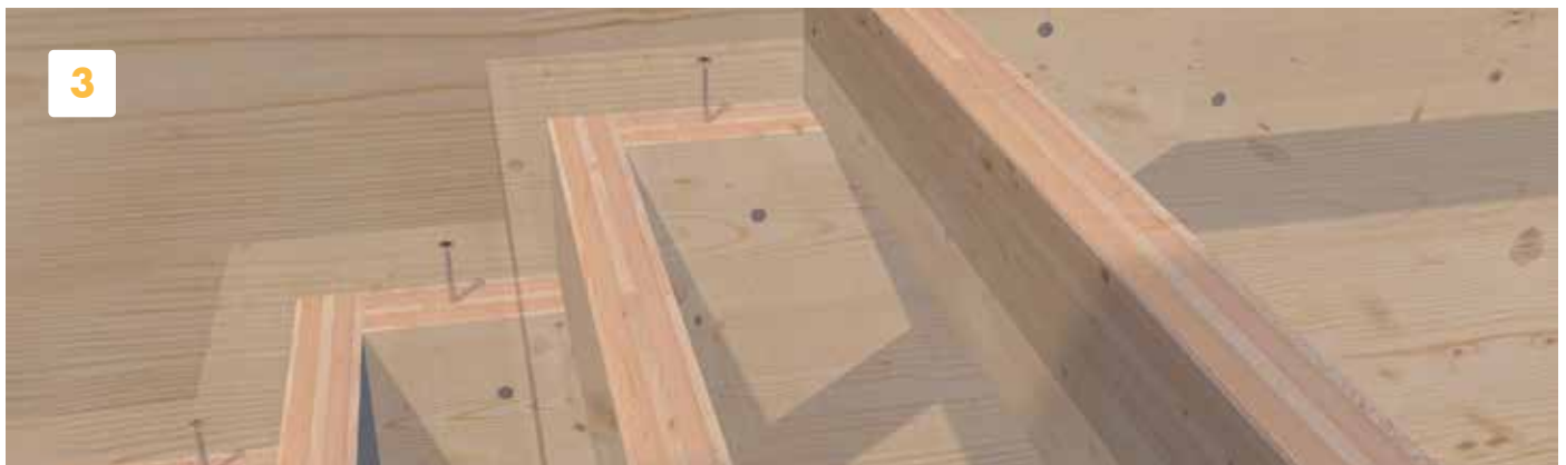
Attach the stair treads on top to the stringer.
